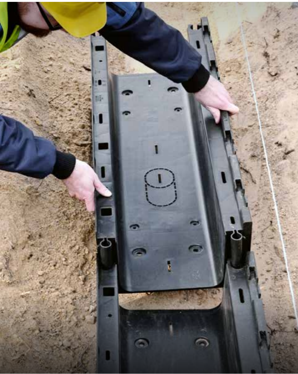
Fig. 1: Connecting of the cable ducts
