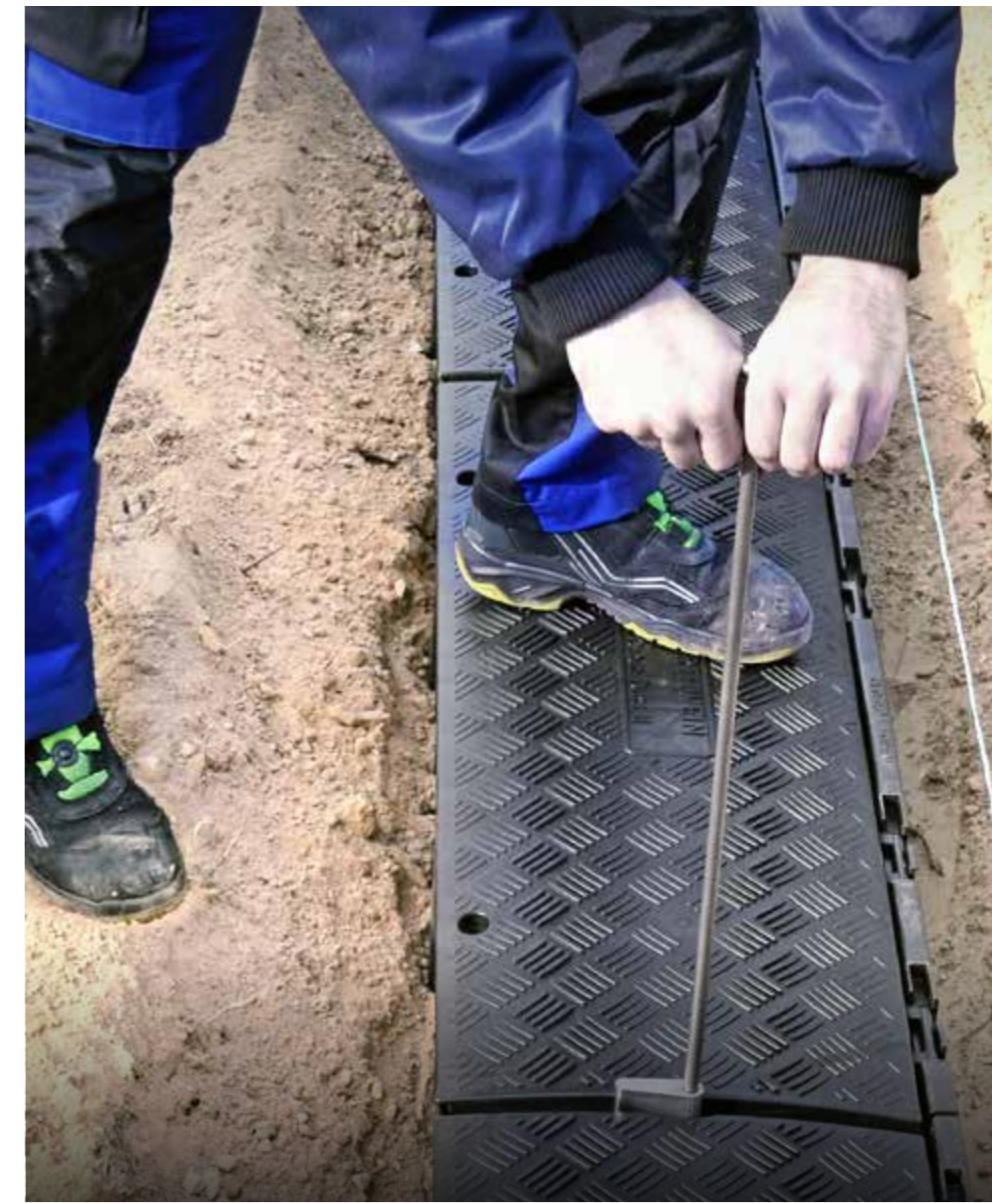
Fig. 3: Locking of the covers
